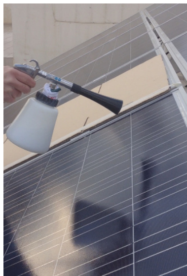
SurfaShield G application with Torna-dor applicator of Bendel.
